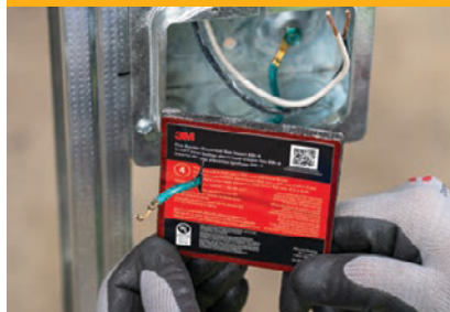
2. Feed wiring through pre-cut slits for easy installation
