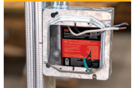
3. Secure insert to the back of the box
