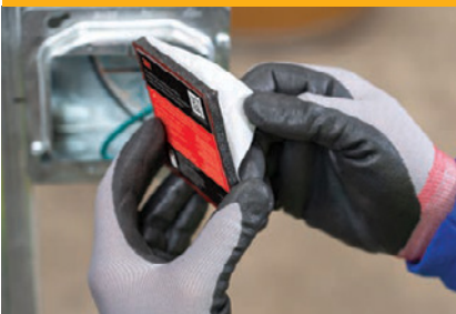
1. Peel off liner to expose the adhesive on the back side of the insert
